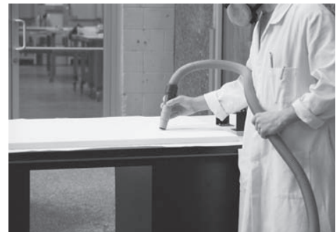
FIGURE 10: VACUUMING DUST FROM THE SHELF AFTER SANDING.
